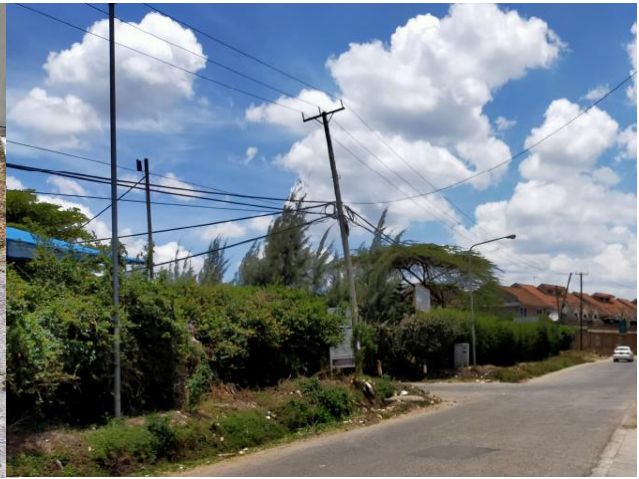
Figure 4-27: KPLC Power lines noted on site
