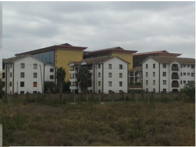
Figure 4-22: Kenya-Re Gardens Estate and KNEC offices in the Background
