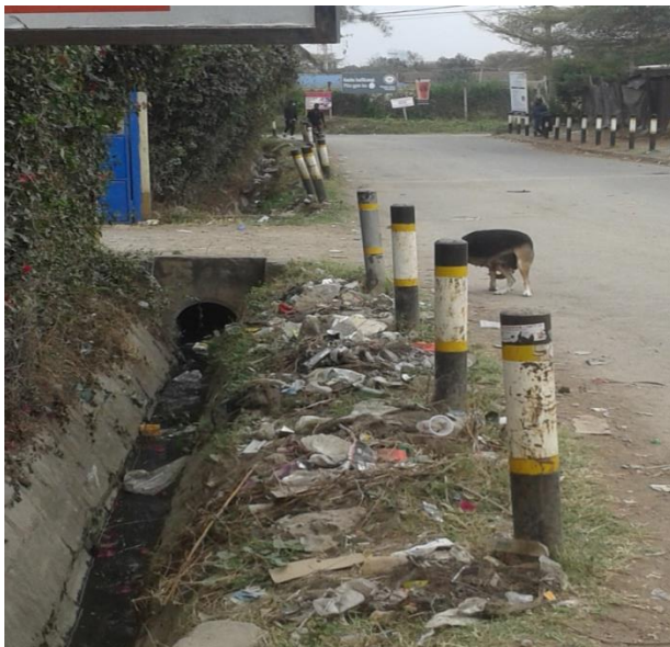
Figure 4-19: Polythene Waste from Storm Drain Opposite Dafam Hotel
