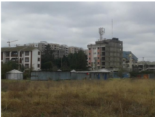
Figure 4-23: Other High rise Buildings Dotting the Skyline at the Project Site.
