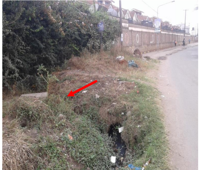
Figure 4-10: Channel draining water from Kenya Assemblies of God Compound
