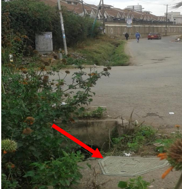
Figure 4-15: One of the Manholes just opposite the gate cited to overflow
